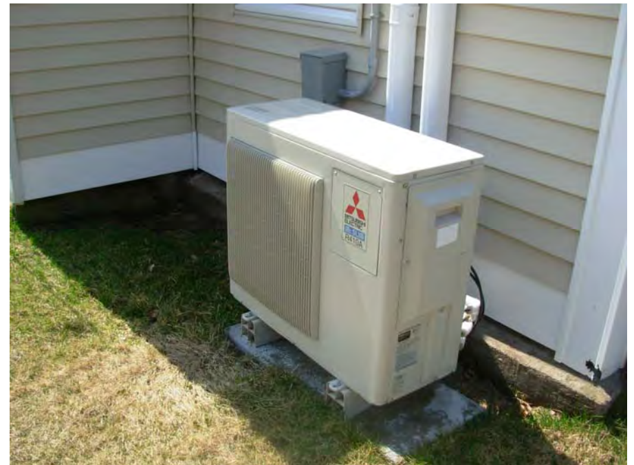
16. Heat pump HVAC system exterior condensers
