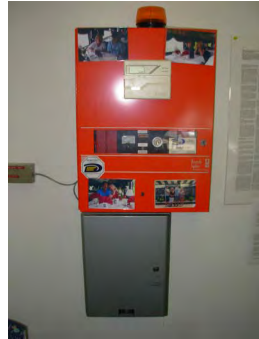
10. Fire and emergency call monitoring panel, in office
