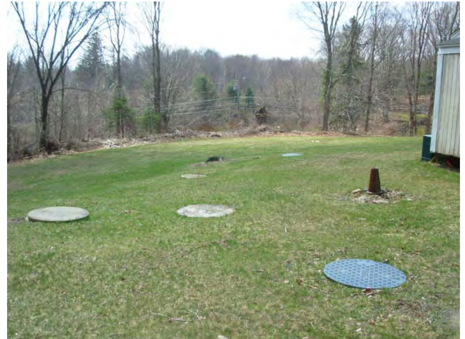
4. View of the septic tank access hatches and leaching chambers beyond
