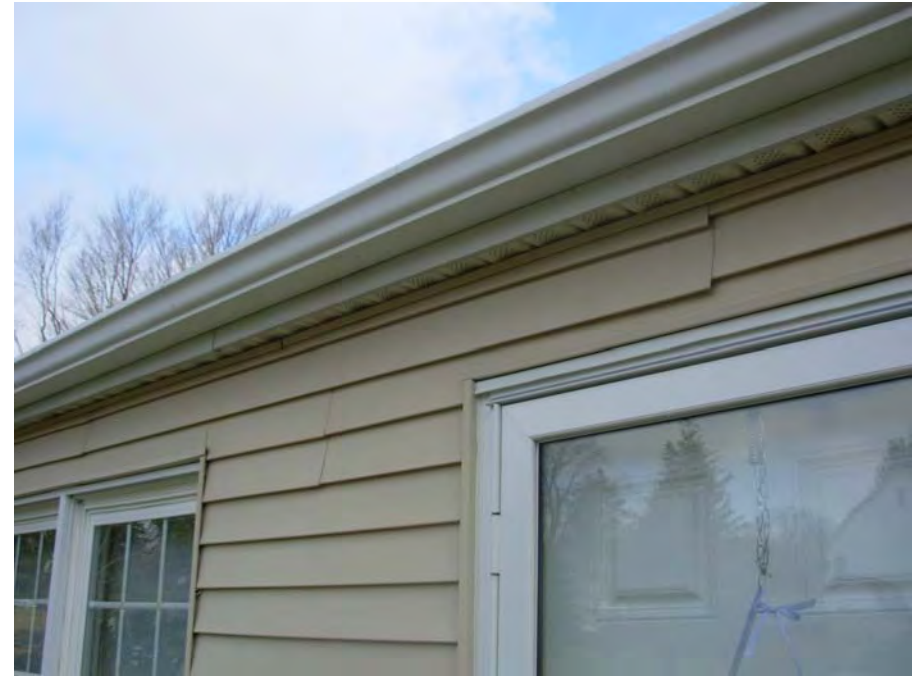
6. Minimal vinyl siding damage
