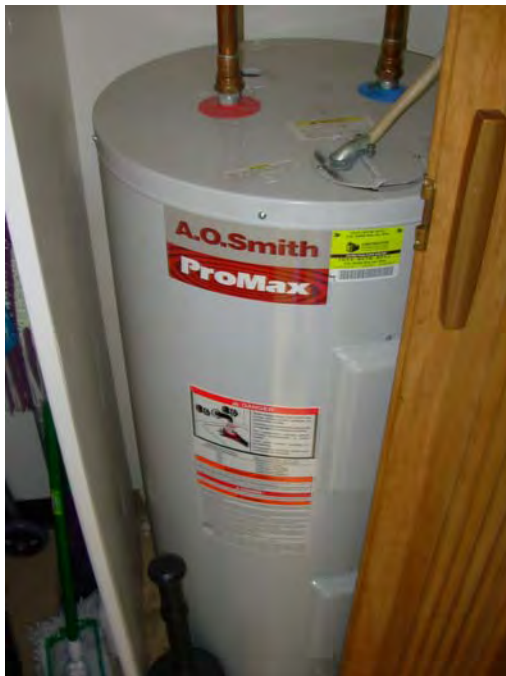
15. Electric DHW tanks serving units
