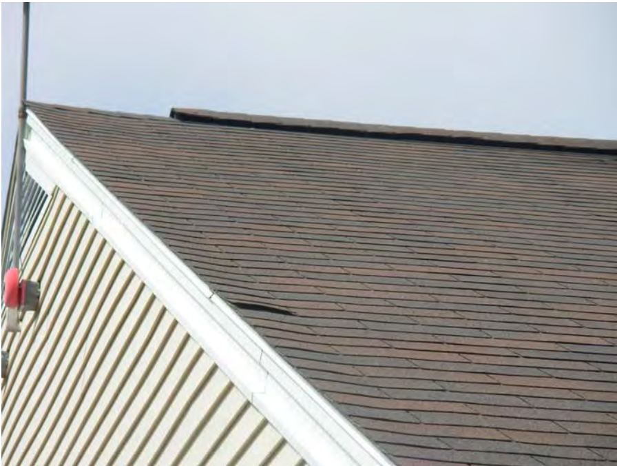
7. Spot roofing shingles lifting, some staining
